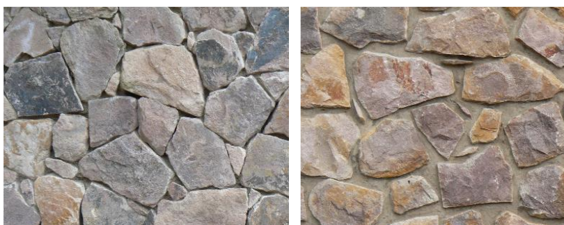
Fig 10, 11: Dry stack and mortar jointed natural stone samples.
